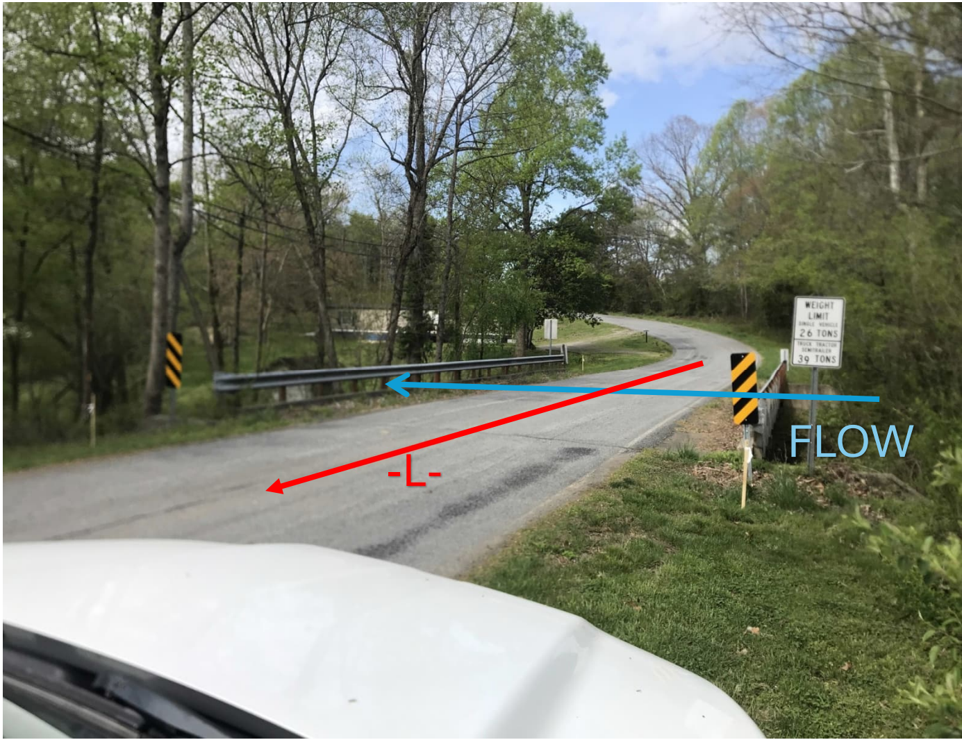
View to west from End Bent 2 towards End Bent 1
